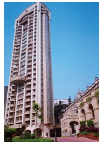
PETIT TOWERS - MUMBAI
