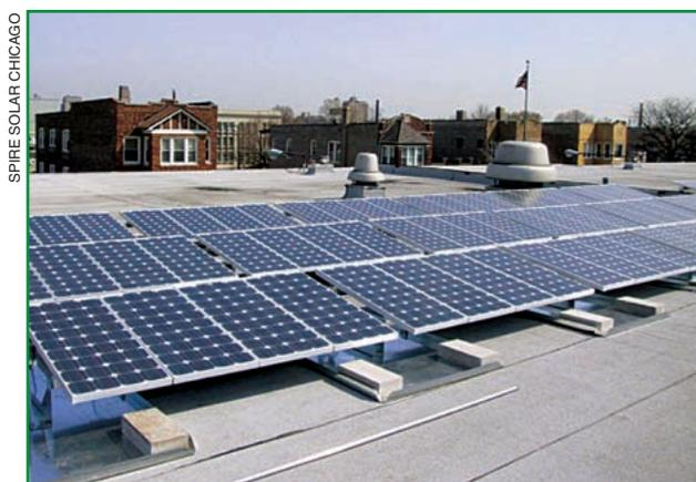
**figure 3.** E. Franklin Frazier Elementary School 10-kW solar PV system.
