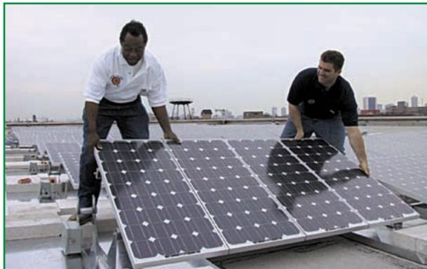
**figure 7.** Electricians from the International Brotherhood of Electrical Workers and National Electrical Contractors Association installing the 38-kW system on the 911 Center.
