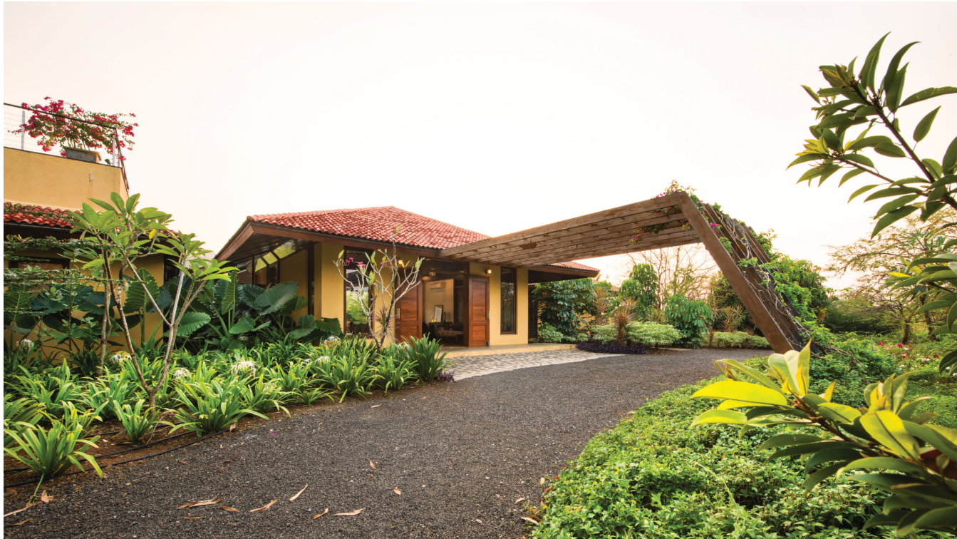
Top: View of Entry Portico
