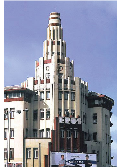
Top L+R: Views of main tower and lantern R: Lantern post restoration
